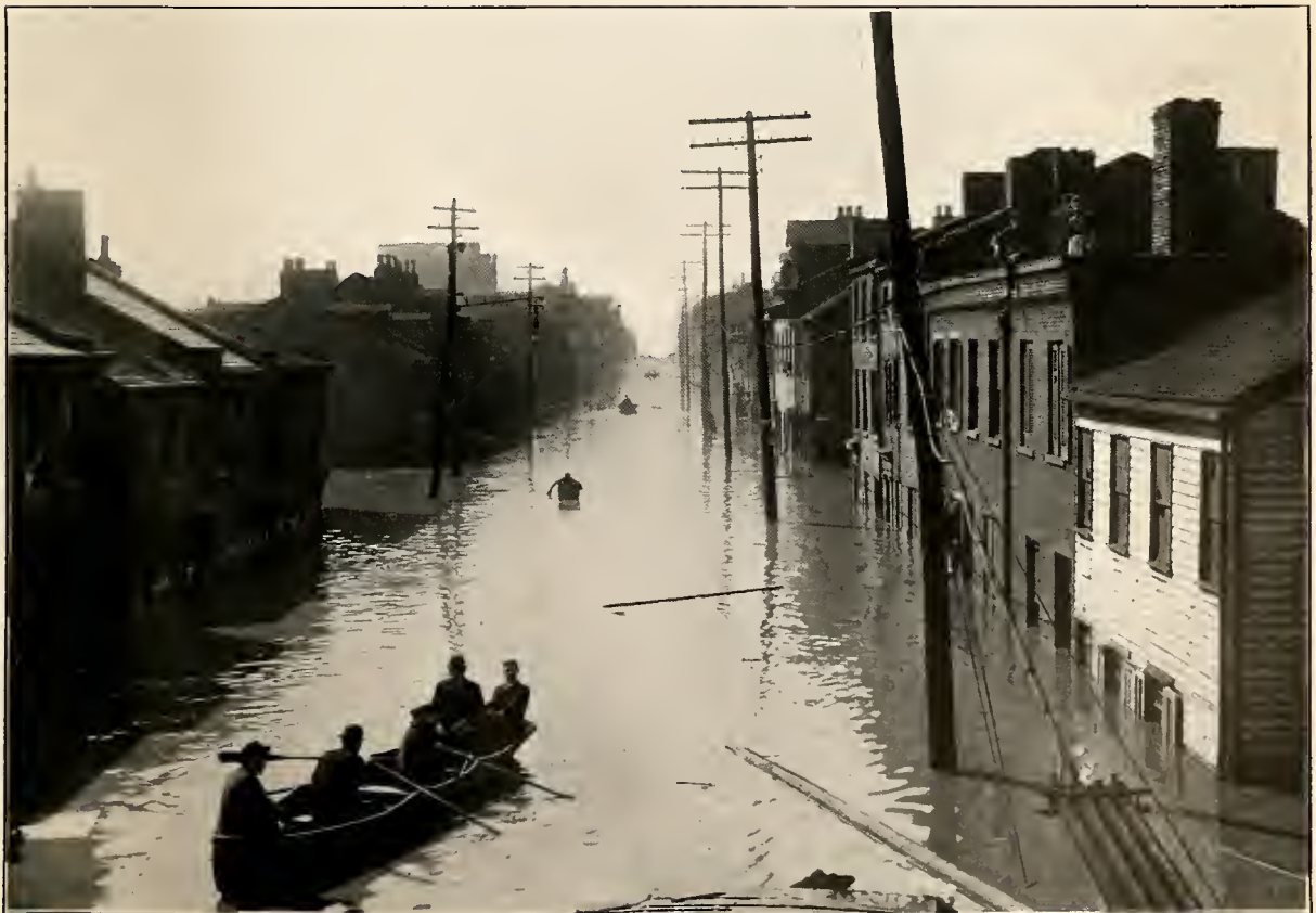
FLOOD OF MARCH 15, 1907. Robinson Street, N. S., looking west from P. F. W. & C. Ry.
